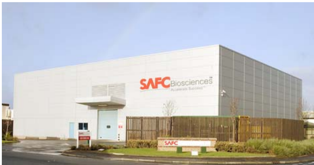
The Facility—courtesy of SAFC Irvine
