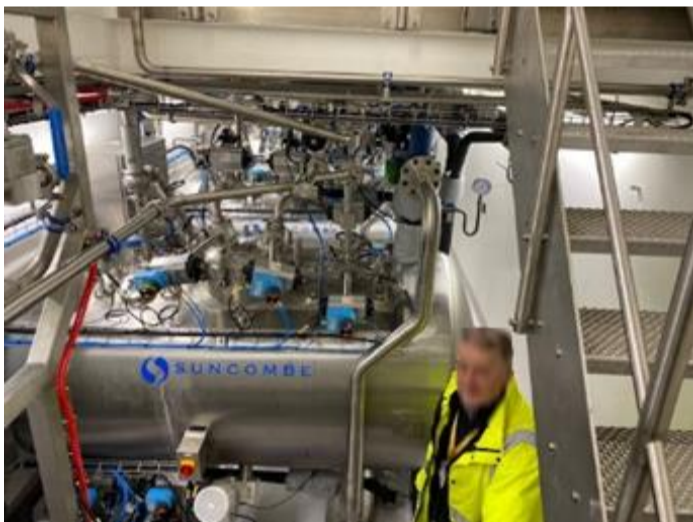
Treatment Hall Entrance
